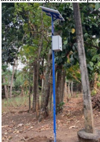
Figure 4 Installation of LEWS Equipment
