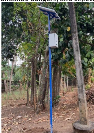
Figure 4 Installation of LEWS Equipment
