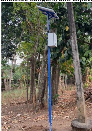
Figure 4 Installation of LEWS Equipment
